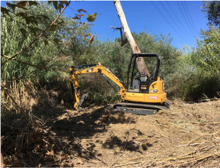
Mini-excavator to Break Clumps
