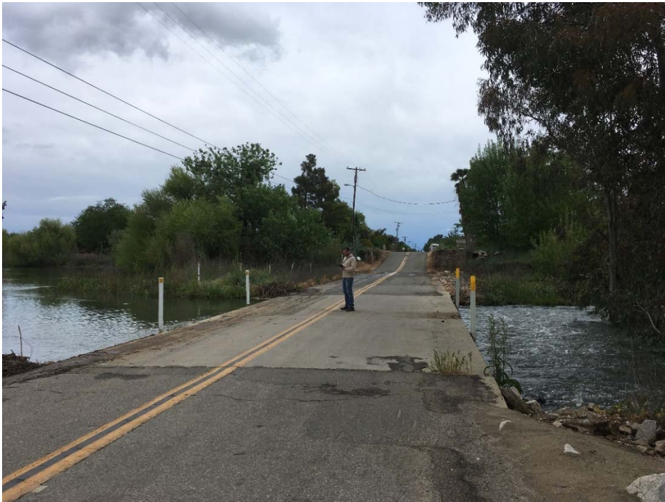
Figure 5-2. River Road Bridge on the Santa Ana River in southern California, pushed off its foundation by floodwaters in 2004 when Arundo biomass lodged against it. Photo by Richard Zembal.
