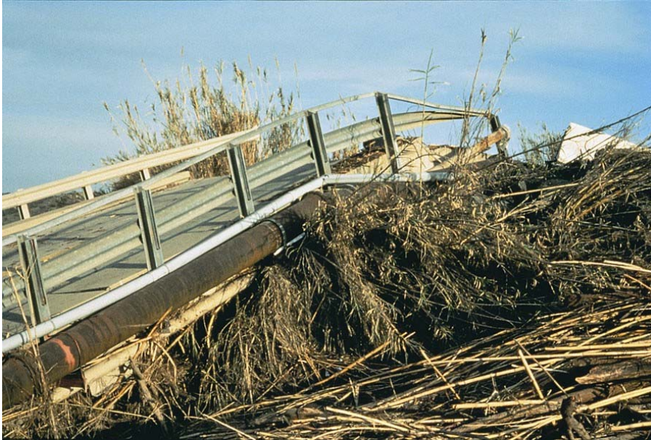
Figure 5-2. River Road Bridge on the Santa Ana River in southern California, pushed off its foundation by floodwaters in 2004 when Arundo biomass lodged against it. Photo by Richard Zembal.
