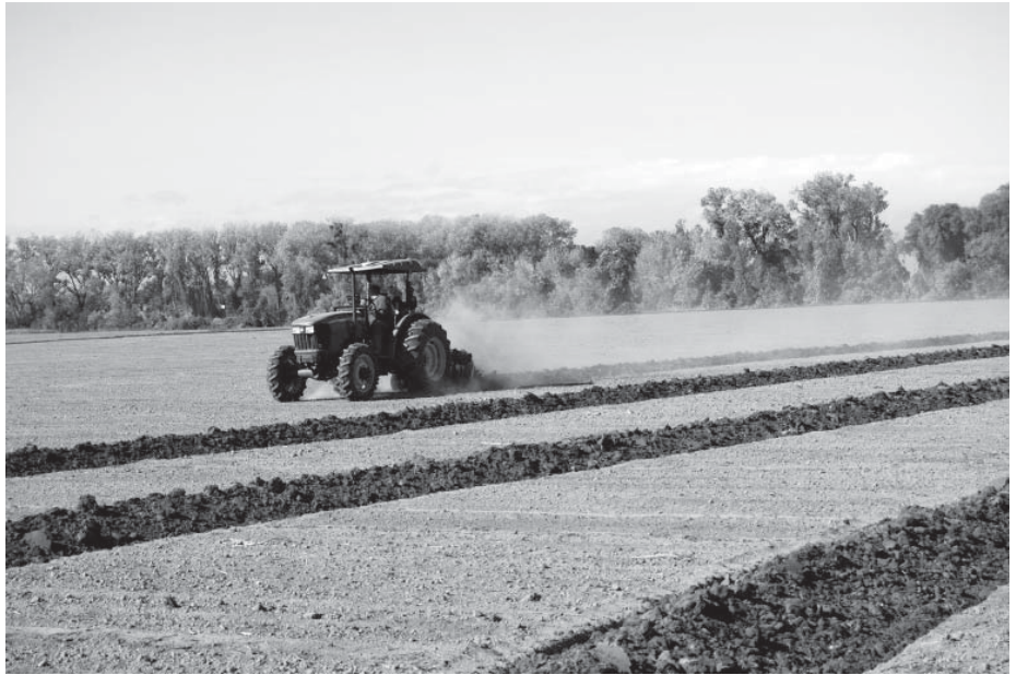
“Pulling” planting berms on a restoration project to prepare for the planting of woody trees and shrubs during the first year of the project.
