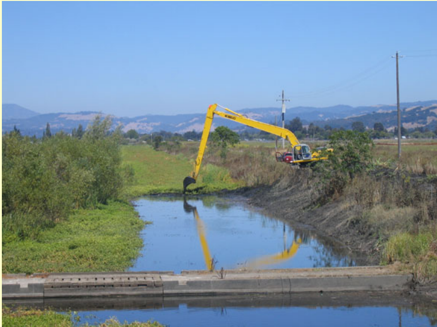
Long Reach Excavator
