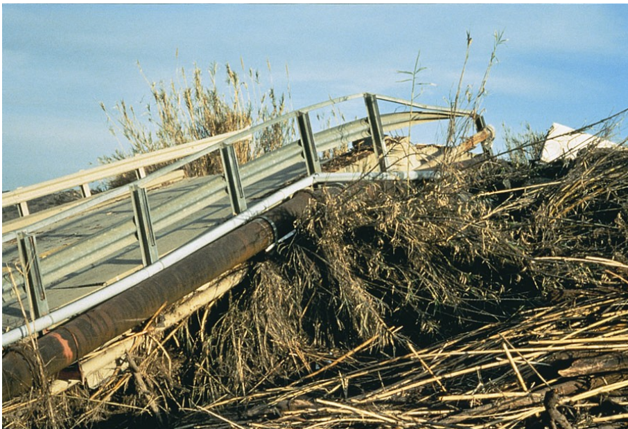
Figure 5-2.29. Floods stacked Arundo biomass against the River Road Bridge on the Santa Ana River, resulting in the bridge being pushed off its foundation in 2004. Photo by Richard Zembal.
