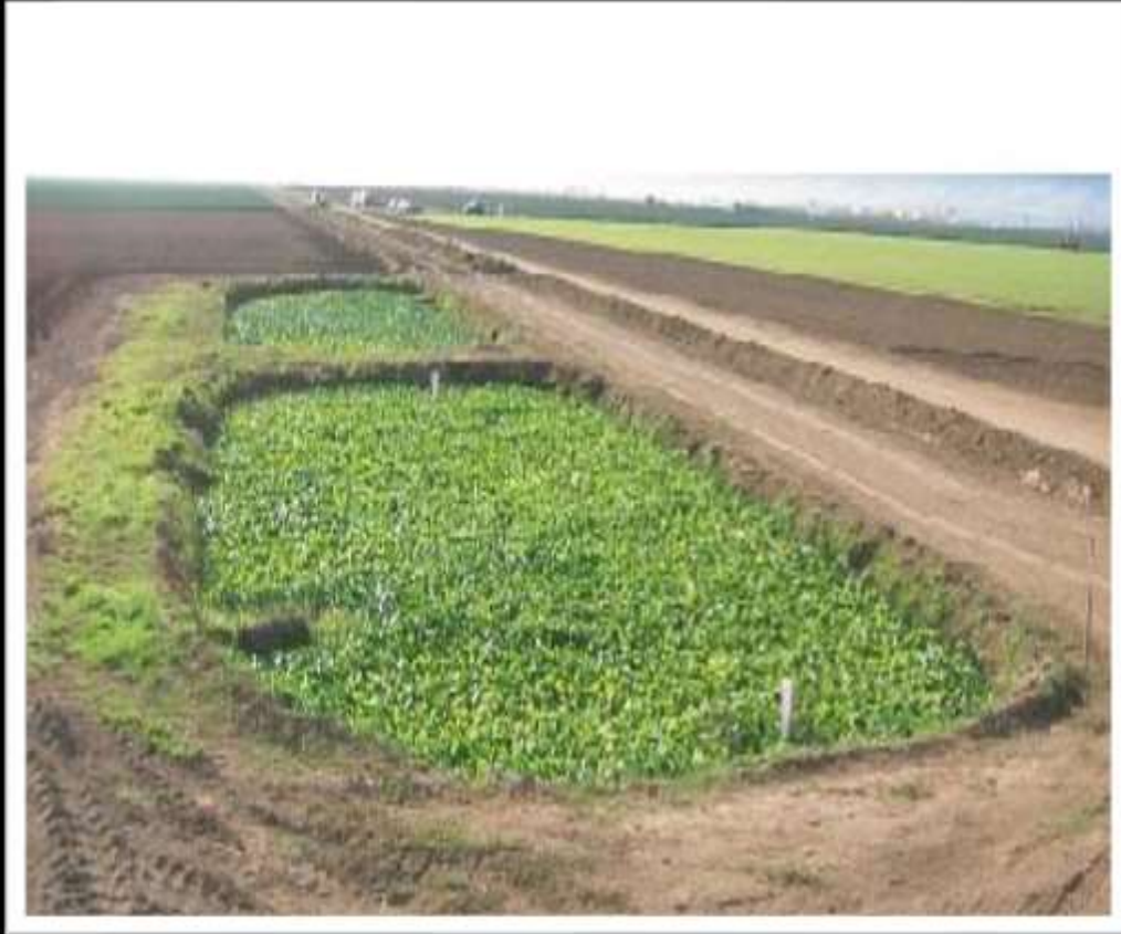
Vegetated Treatment Pond
