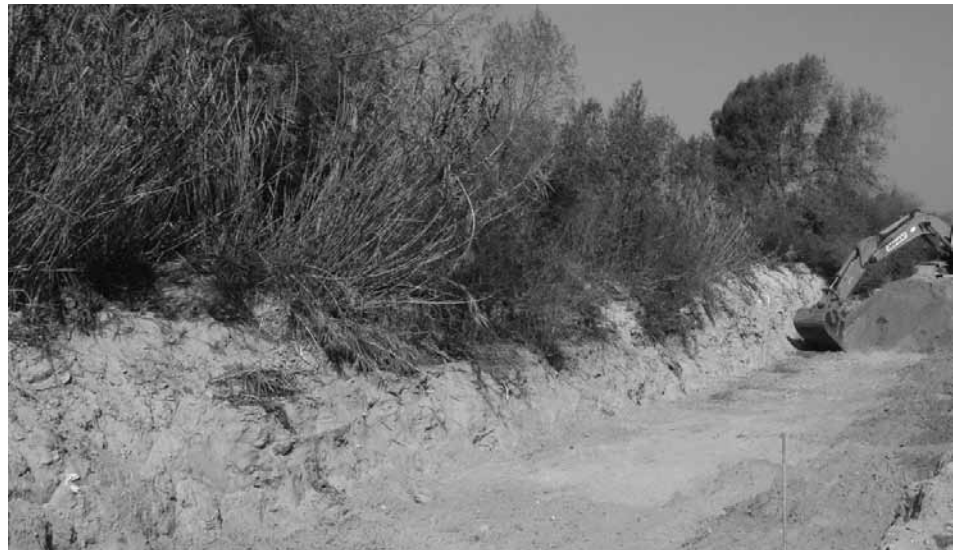
Arundo donax is being unintentionally spread by this backhoe. Simple measures can be taken to prevent mechanical dispersal of arundo.
