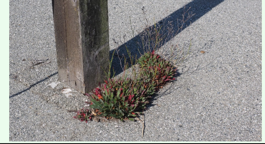
Limonium ramosissimum exploiting a crack in the concrete adjacent to Sanchez Marsh
