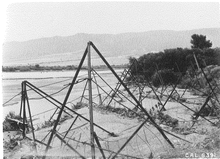
Plate 3. Same site as plate 2 but taken in August, 1942. Note the silt deposition behind the tetrahedrons, and that the area is beginning to be revegetated. Note also settling of the tetrahedrons indicating the unstable condition of the stream channel.
