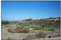
Crews removing biomass, Site 2
