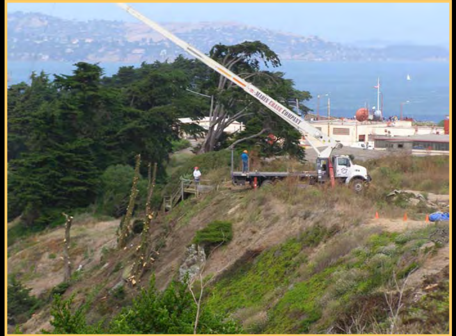
Mattress wire weed and tree removal
