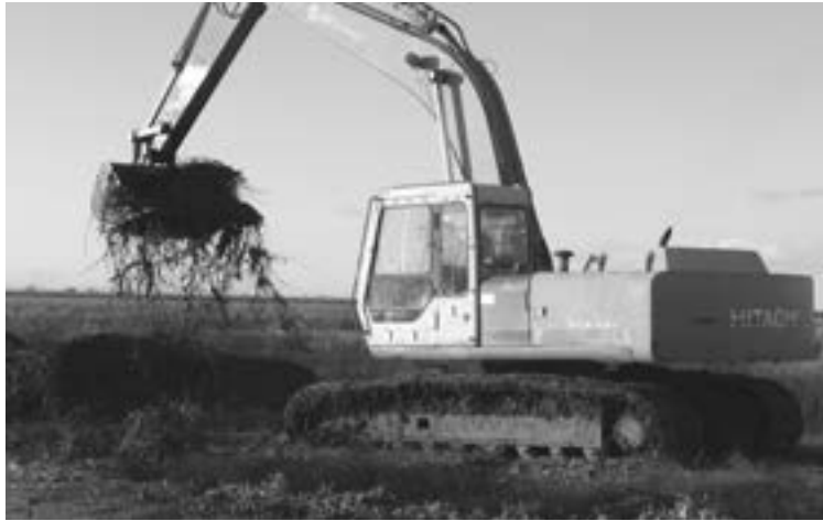
Removing aquatic invasive plants with equipment such as a backhoe must be done in a way that minimizes disturbance. Photo by Joel Trumbo.
